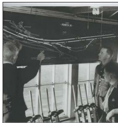
Penrith No.1 Signalling diagram. Allan Beck. On the closure of Redhills Jn. and Eamont Jn. signal boxes in 1938 a new illuminated diagram was provided in Penrith No. 1 to control the expanded area. It looks as though this is a signalman's training session ready for implementation with the white lines showing track circuited lines.
