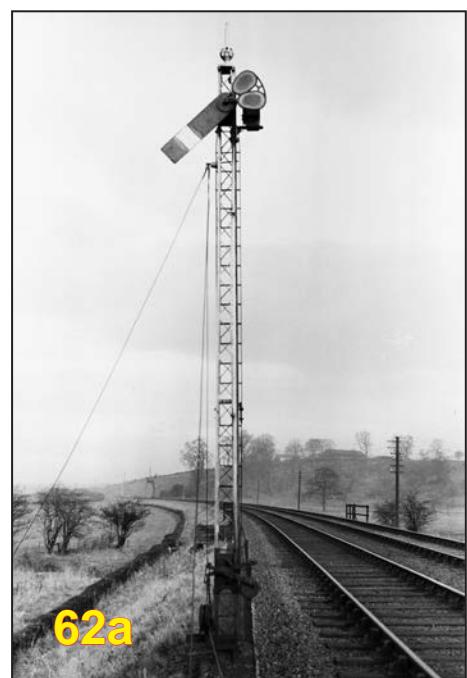
the photos were taken by I Pearsall, with PEF963 showing Cummersdale's Down Starter, which was a M&C type lattice post, whilst PEF966 showed LMS 5MT 4-6-0 45092 on a goods over the viaduct, both taken on 5th February 1955. **Allan Beck** confirmed that the M&C Lower Quadrant signal was the Up Starter (as it was then) and was situated at the very end of Caldew viaduct on the Carlisle side.
