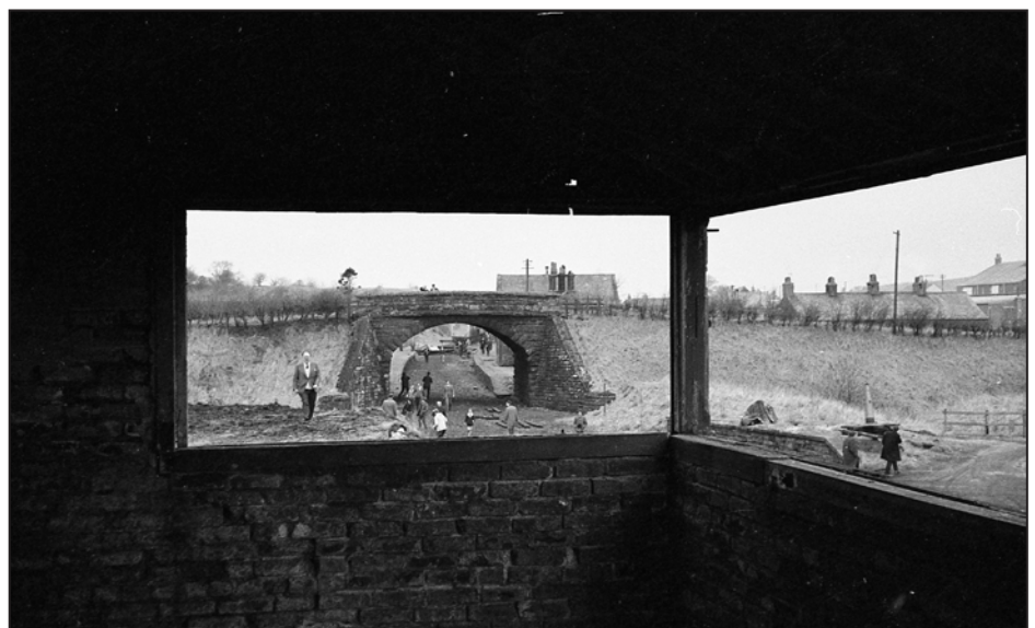
View taken from the redundant signal box whilst Keith Fenwick visited the area on a Railtour in 1969. The photo shows the low arch overbridge which would explain the gallow signal to allow better sighting. Keith Fenwick.
